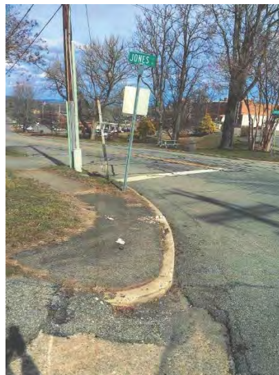
Sidewalk deficiencies in Martinsville include uneven pavement and curb cuts needing repair
