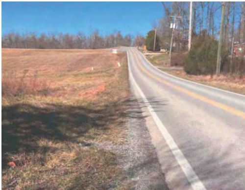
Morewood Rd: No curb, gutter or sidewalk
