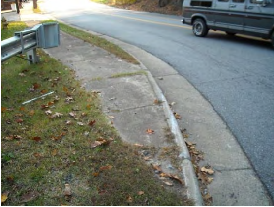
Fairystone Park Hwy: Northeast side from intersection of Trent Hill Dr to bridge across from EMI
