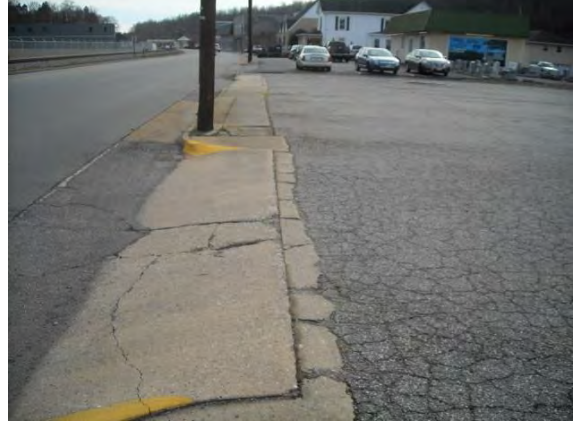
Fairystone Park Hwy: Southwest side east end of bridge going southeast
