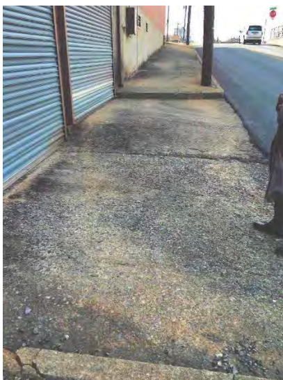
Sidewalk deficiencies in Martinsville include uneven pavement and curb cuts needing repair
