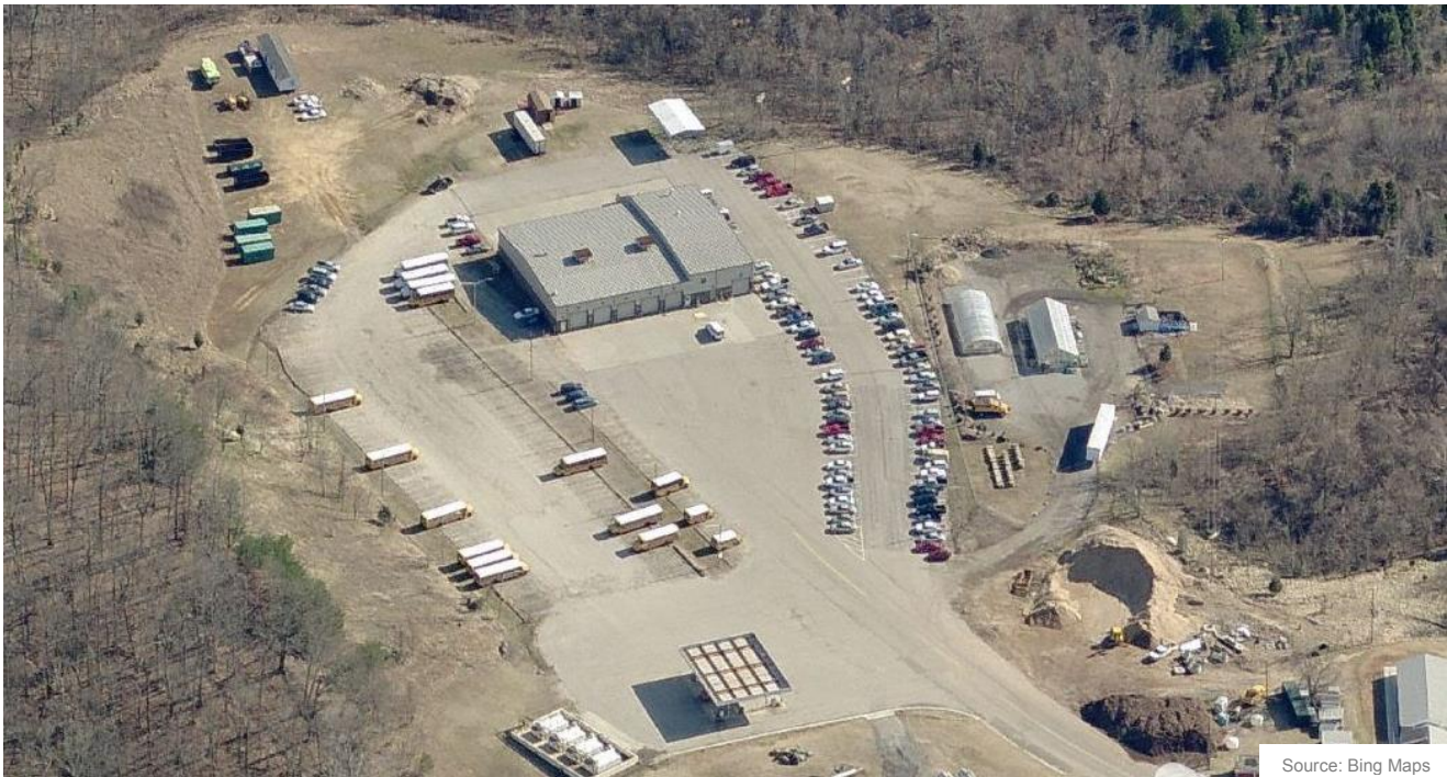
Danville Transit’s Administrative and Maintenance Facility
