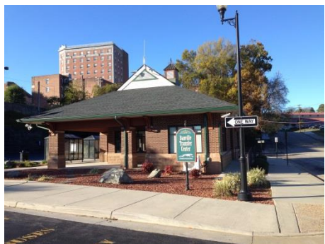
Danville Transit Center downtown "HUB"
